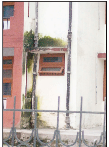
The effects of seepage taking toll of newly constructed tenements at Jagti. --KS photo
