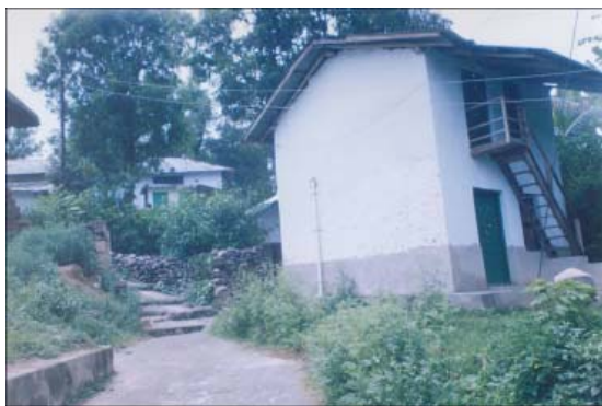
A new house (with wooden staircase) on the land, where once stood the ancestral house of Suresh Raina, Test Cricketer. The house had collapsed a few years back and the property was sold by Suresh Raina's family.
